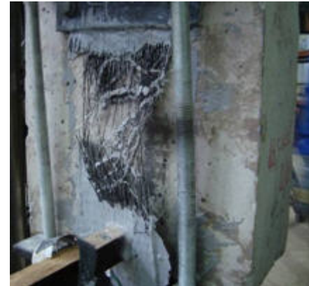
Fig. 6c. Tensile failure of the FRP strip
