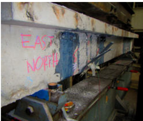
Fig. 13. Debonding of the open hoop CFRP strips at the East part of the T-Beam
