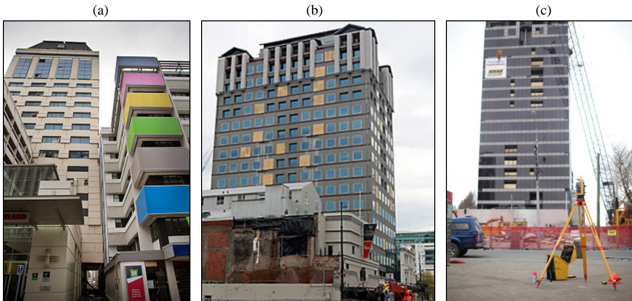
Fig. 3 – Buildings damaged during the 2010 – 2011 Canterbury earthquake sequence that were subsequently demolished: (a) Hotel Grand Chancellor 1 ; (b) Clarendon Tower 2 ; (c) PricewaterhouseCoopers building 3
