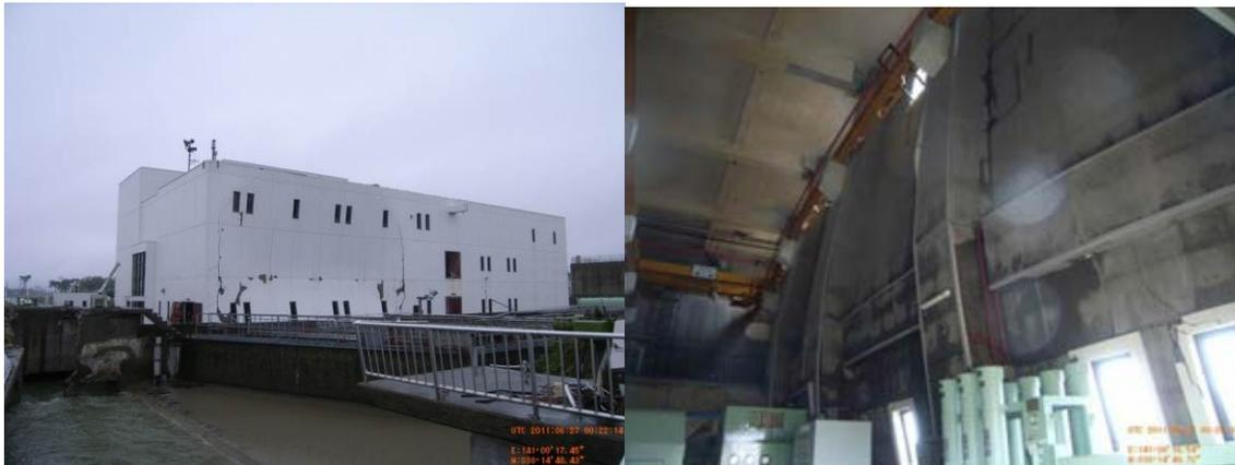
Fig. 6 - Ocean-facing reinforced concrete wall at the Minami Gamou Wastewater Treatment Plant pump station building damaged by direct strike from tsunami bore (a) exterior view, (b) interior view
