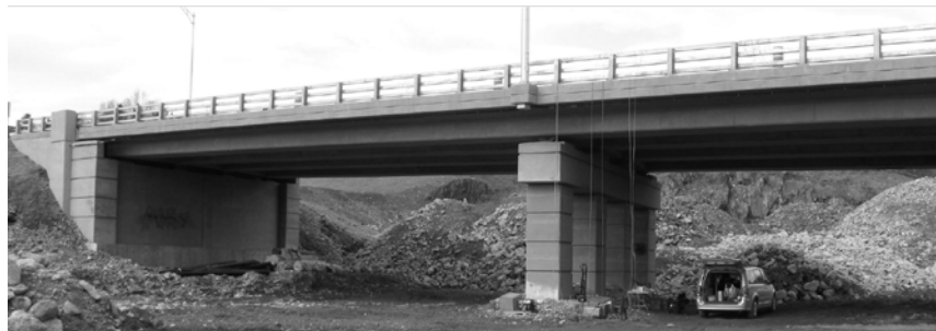
Fig. 1 – Bridge 1 (over future Highway), built in 2011
