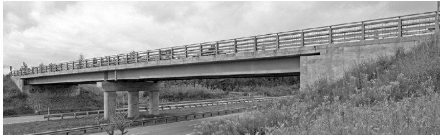
Fig. 3– Bridge 2, over four lane highway, built in 2010
