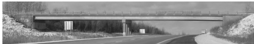
Fig. 5– Bridge 3, over four lane highway, built in 1977
