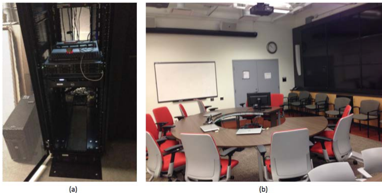
Fig. 5 – Seismic monitoring control room at the UBC
