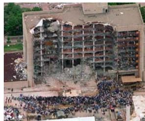
Fig. 1 – AP Murrah Building Progressive Collapse
