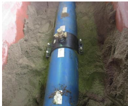
Picture 4 – Pipe with a branch saddle (200 A)
