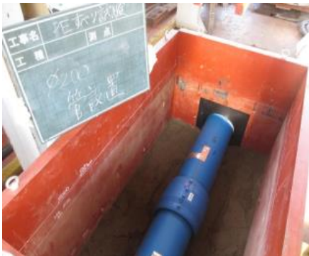
Picture 3 – Pipe with EF coupler (200 A)
