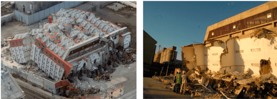
Fig. 1 – Building 1 after the February 27, 2010 earthquake in Chile
