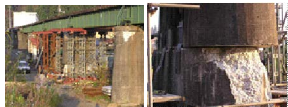
Fig. 1 – Uonogawa Bridge damaged during the 2014 Niigata-ken Chuetsu Earthquake [3]
