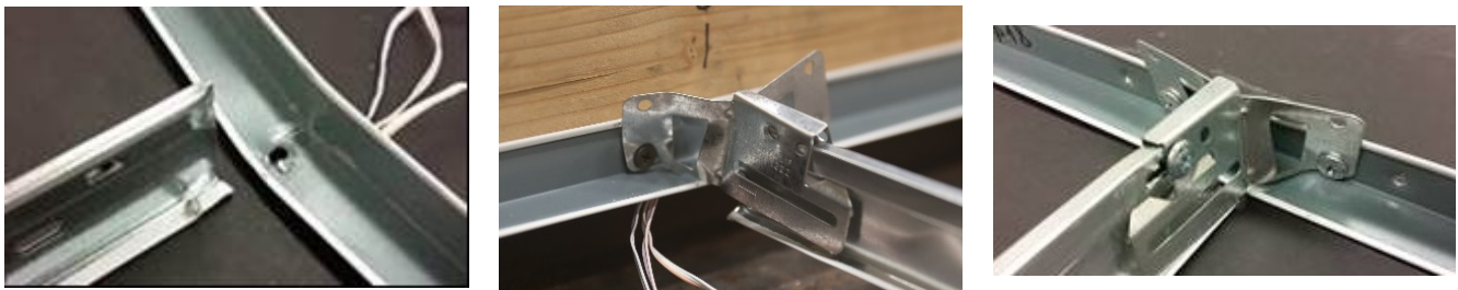
Pop riveted connection
