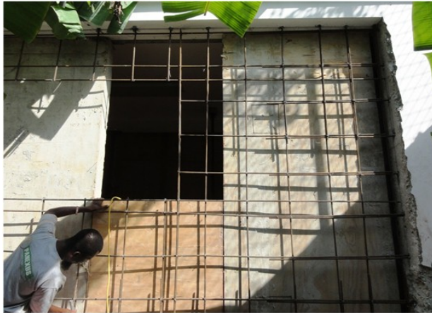
Addition of new shearwall
