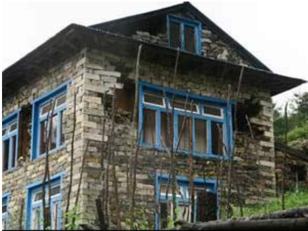
Fig. 9 Out-of-plane failure of bearing wall building
