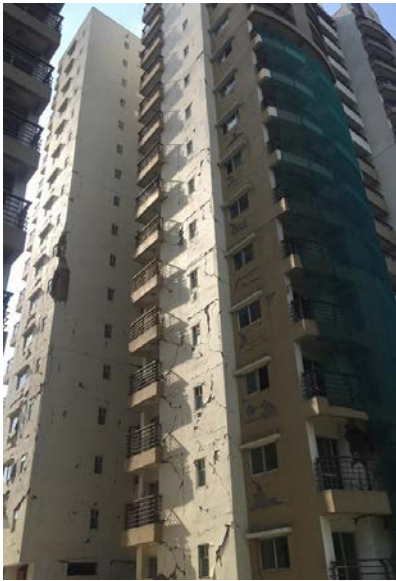
Fig. 11 Exterior cracking, residential tower
