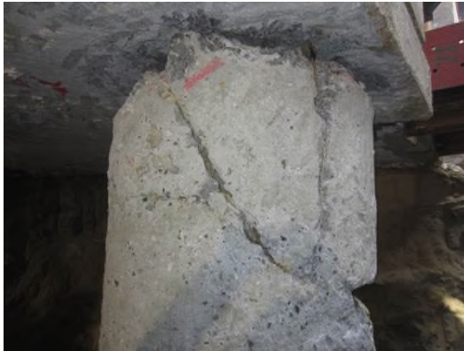
(a) After removing surface concrete (D-7)
