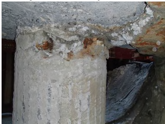
(c) Damage of cover concrete at pile head (D-5)
