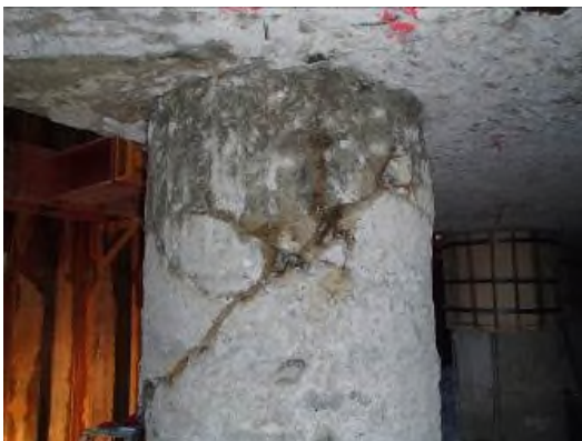
(a) After removing surface concrete (D-7)
