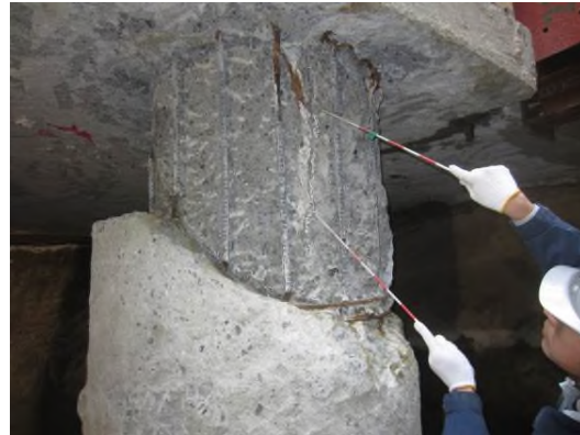
(b) After removing cover concrete of pile head (D-7)
