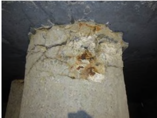
(a) Damage of cover concrete at pile head (A-6)
