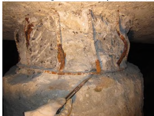
(d) After removing cover concrete of pile head (D-5)
