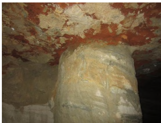
(a) After excavating (Location; B-5)
