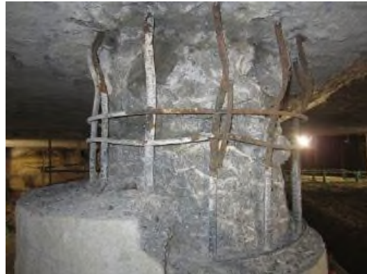
(b) After removing cover concrete of pile head (A-6)
