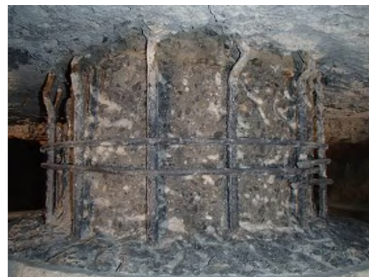
(d) After removing cover concrete of pile head (B-5) Local buckling of main rebar at pilehead joint
