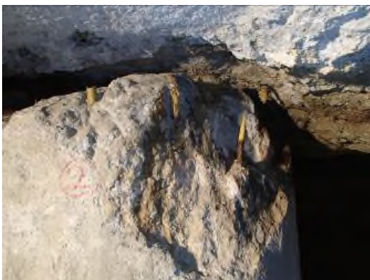
(a) After removing surface concrete (Z-5)
