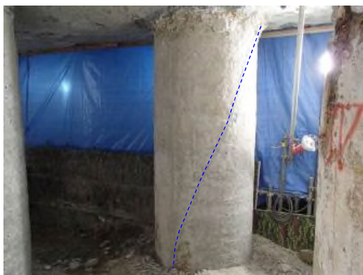
(a) After removing surface concrete (C-4)
