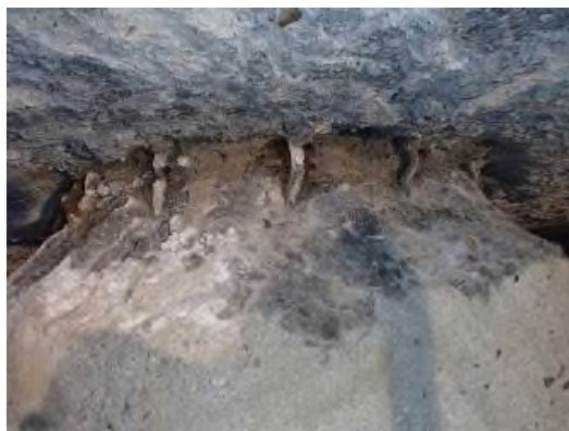
(c) After removing fragile part of concrete (B-5)
