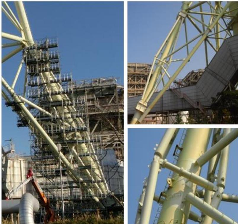
Photo 2 – Pantograph-type response control system
