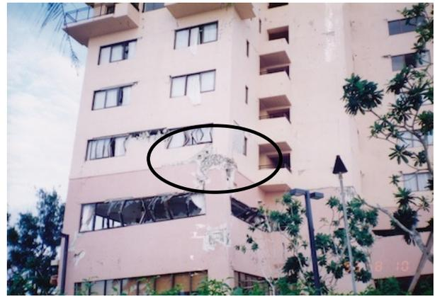
Fig. 1 – Joint hinging model at exterior joint [2]
