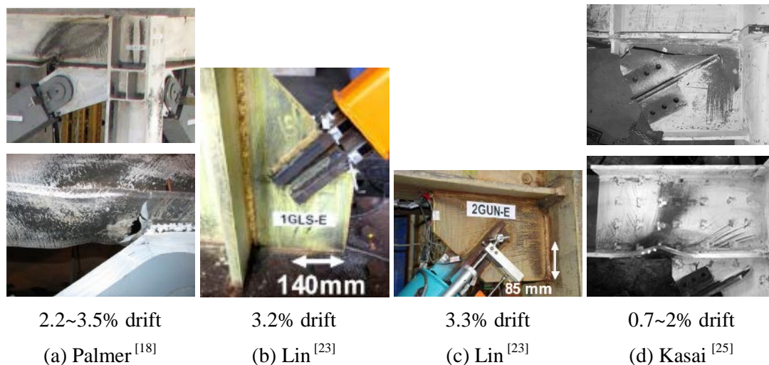
Fig. 9 – Damage to adjacent framing and gussets due to in-plane drift
