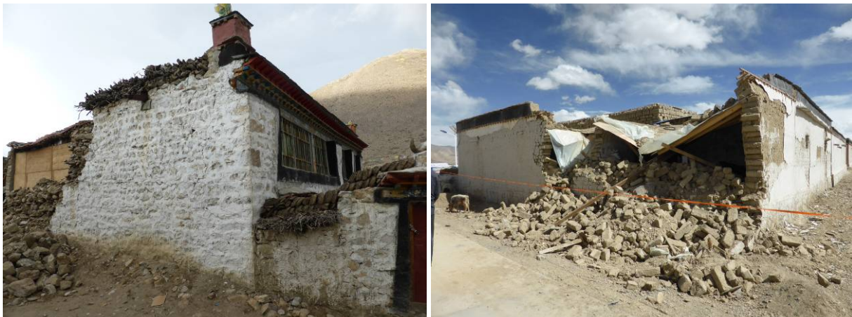
Fig.12 – Collapsed rubble building (left) and soil building (right) in Tibet
