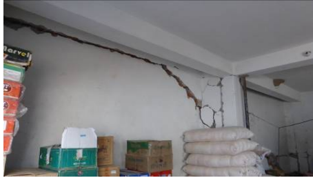
Fig. 5 –Serious damaged RC houses in Deupur
