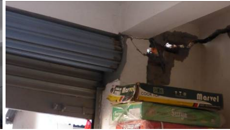
Fig. 5 –Serious damaged RC houses in Deupur
