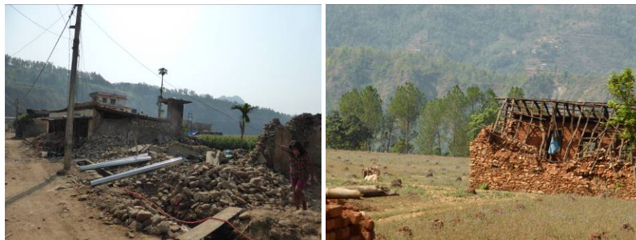
Fig. 4 – Collapsed rubble houses in Deupur (left) and Necpane (right)
