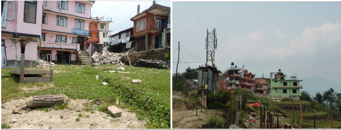
Fig. 9 – Several RC buildings collapsed due to the ground instability
