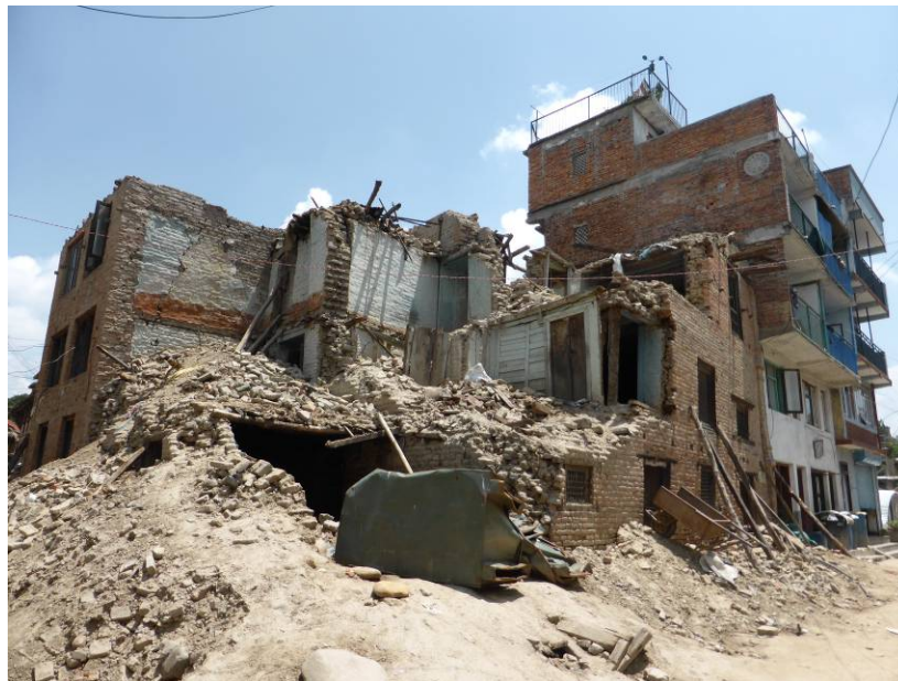
Fig. 6 – Collapsed brick-wood houses in Kathmandu
