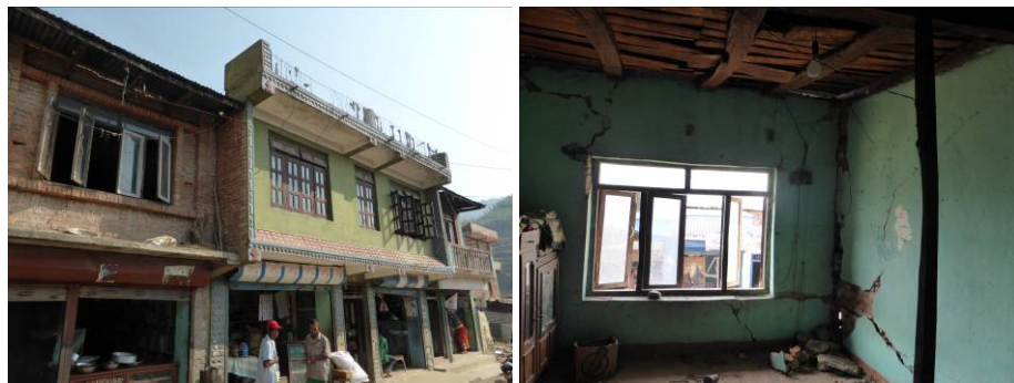
Fig. 3 – Serious damaged brick-wood house in Deupur
