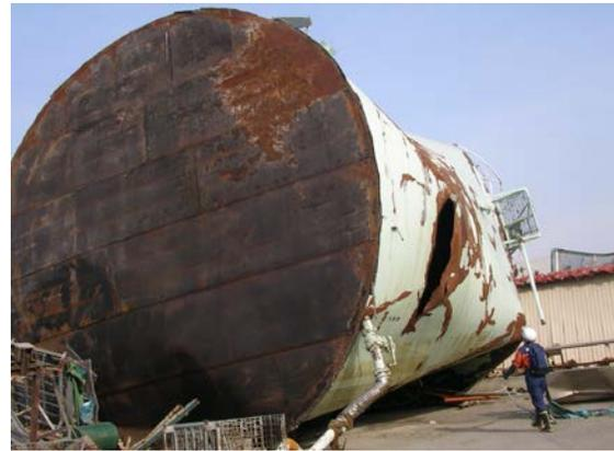
Fig. 1 – Oil storage tanks moved by tsunami in Kesenuma City, Miyagi Prefecture. (Images taken by Dr. Kiminori Araiba of NRIFD on April 7, 2011.)
