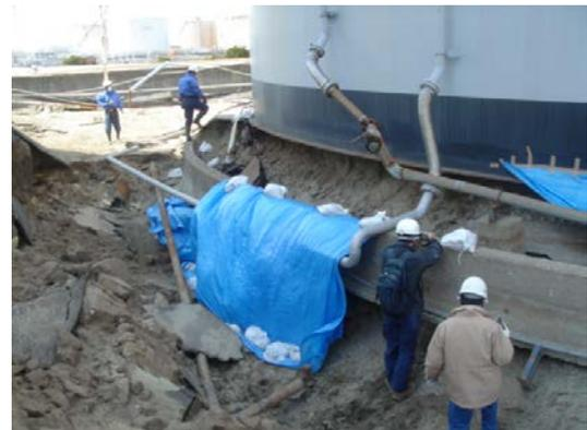
Fig. 3 – Tank base and ground scoured by tsunami in Sendai City, Miyagi Prefecture.
