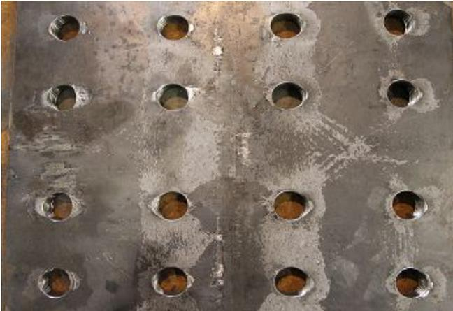
Fig. 7 – Damage in flange splice plate
