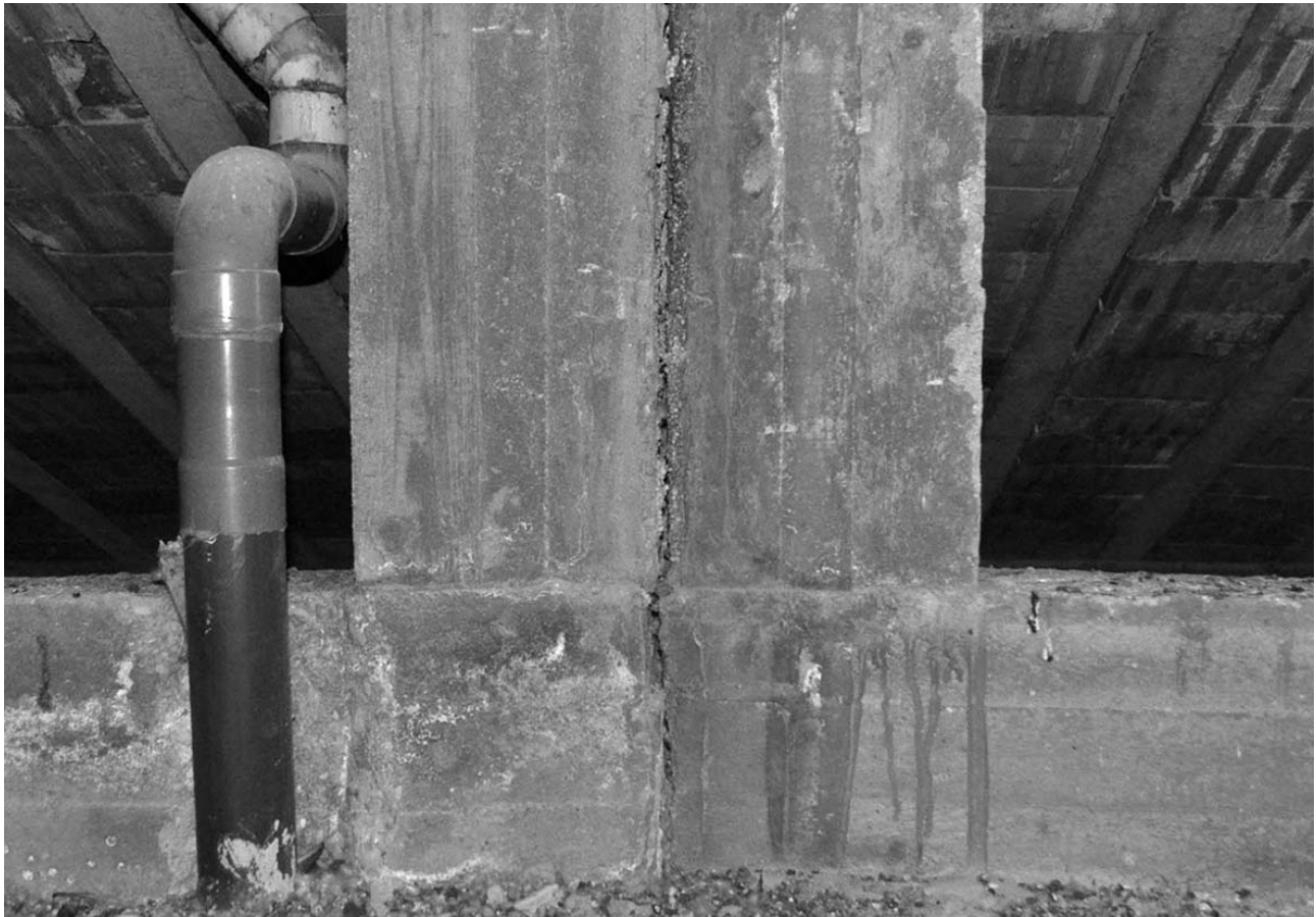
Fig. 6 - The joint between the two monitored blocks
