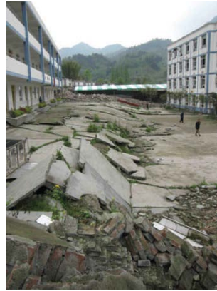
Fig. 6(b) - Fault Rupture through a School at Bailu
