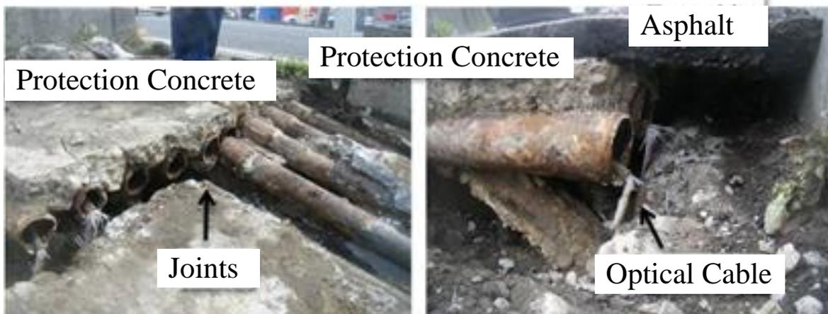
Fig-1: Damage to optical-fiber cable after the Great East Japan Earthquake
