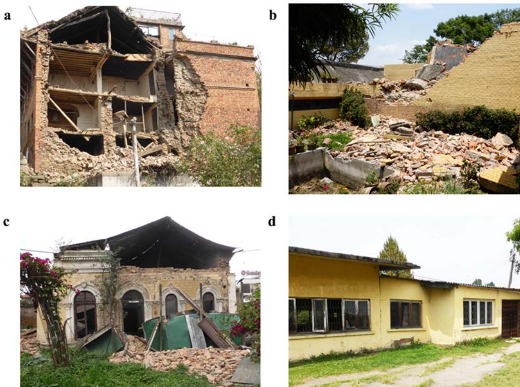
Figure 7 – a) Collapsed facade in KTP, b) Damaged masonry building in TVU, c) Damage to masonry building with ' bajra ' mortar, and d) Damaged school building in THM.
