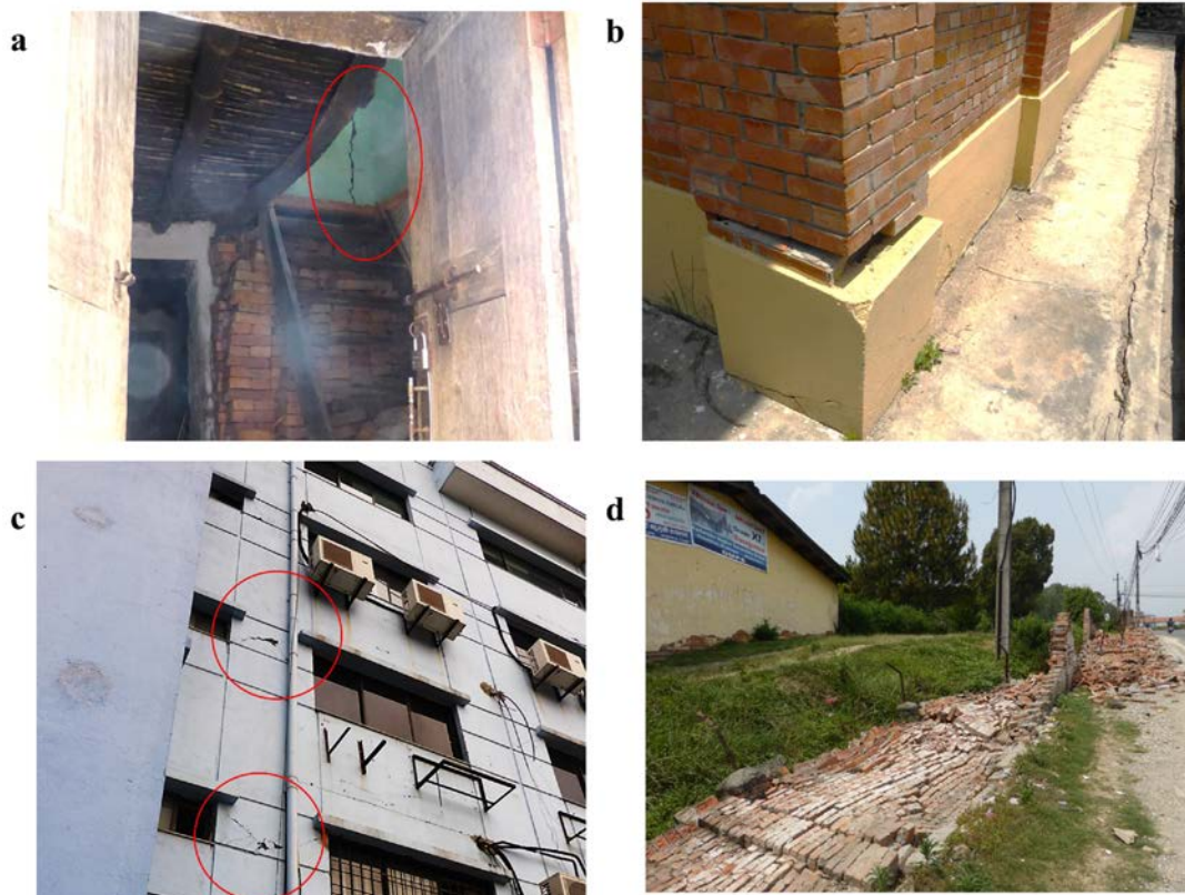
Figure 6 – a) Cracks developed in masonry buildings of KTP, b) Damaged columns in ground floor of a RC buildings at TVU, c) Shear-cracks seen in a RC building in PTN, and d) Collapsed compound wall in THM.
