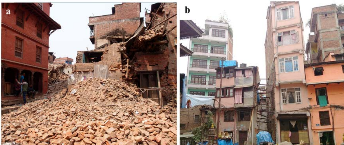
Figure 4 – a) Loss of mud-mortar from the fired-bricks in Bhaktapur, b) Asymmetrical designs of RC building in Kathmandu taken before the earthquake.
