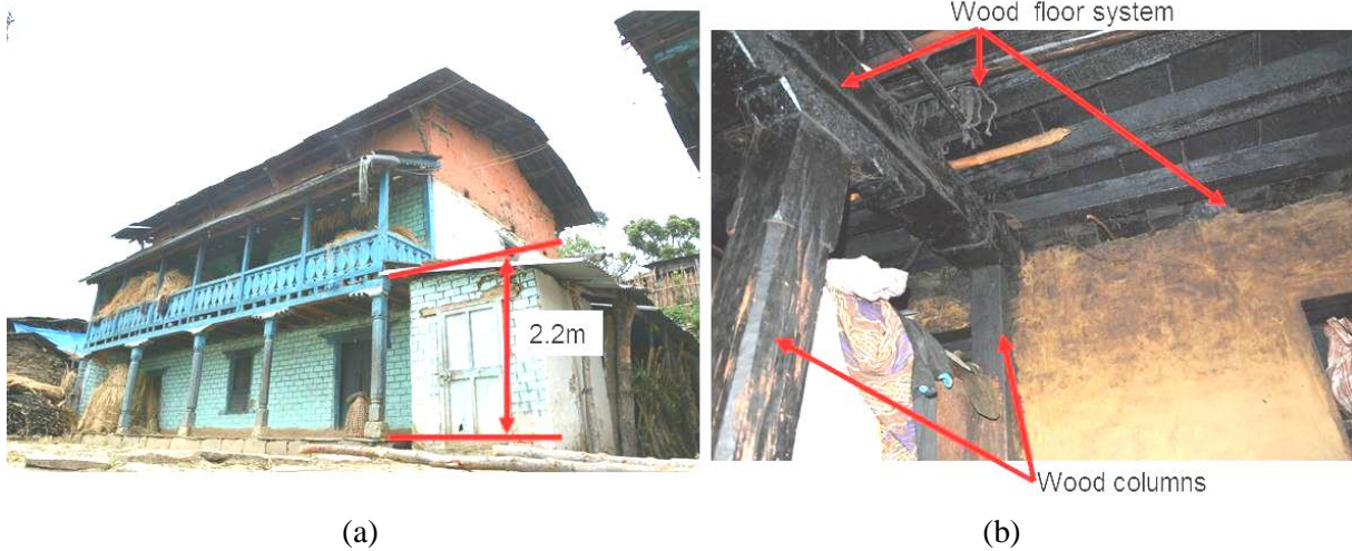
Fig. 3 – Wood strengthened stone-soil structure (at Pangdang, a village in Sindhupalchok District)
