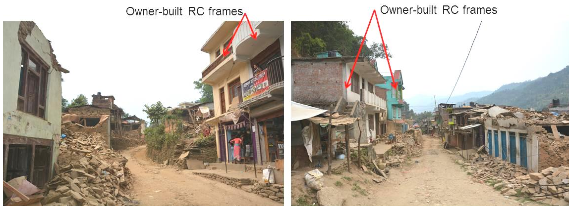
Fig. 2 – Difference of damage degree between various types of structures (at Jalbire, a village in Sindhupalchok)
