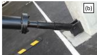
Figure 8. Viscous devices implementation (Google Maps and MacRae) Figure 9. CBF Application (MacRae)
