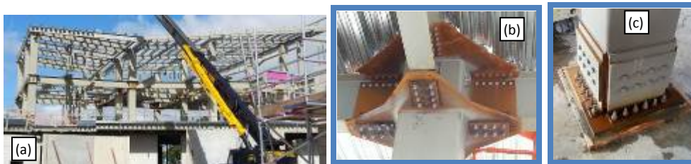
Figure 6. Details of the Friction Connections on the Terrace Project (MacRae)
