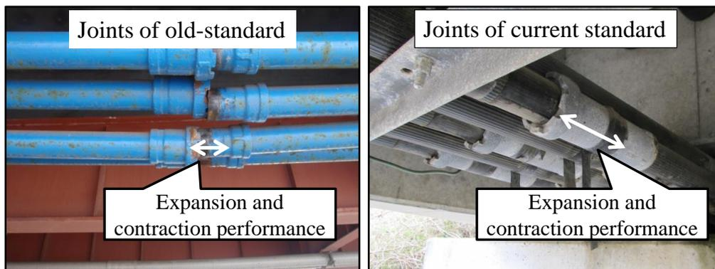
Fig. 3– Joints of old-standard and joints of current-standard
