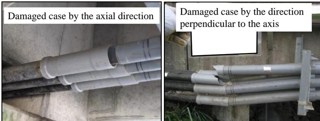
Fig. 2– Examples of damage mode
