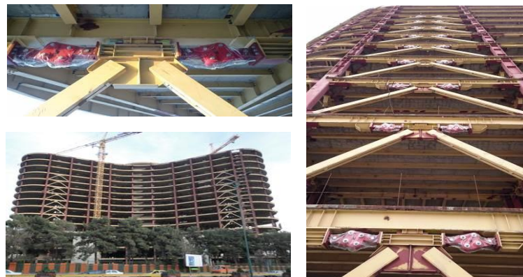
Figure 20 - Dampers installed in large hospital project.
