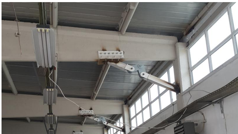
Figure 22 – V-shaped rotational friction dampers on precast RC structure
