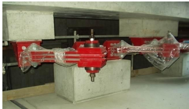
Figure 13 - Three residential towers with RFDs Figure 14 – Dampers installed in residential tower in Osaka, Japan
