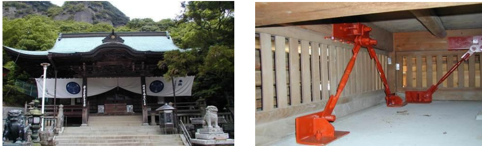
Figure 6 – Dampers with bracings installed in Yagutji Temple
