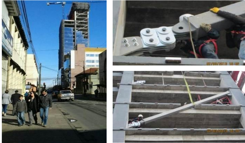
Figure 21 - Dampers installed in diagonal bracing system.
