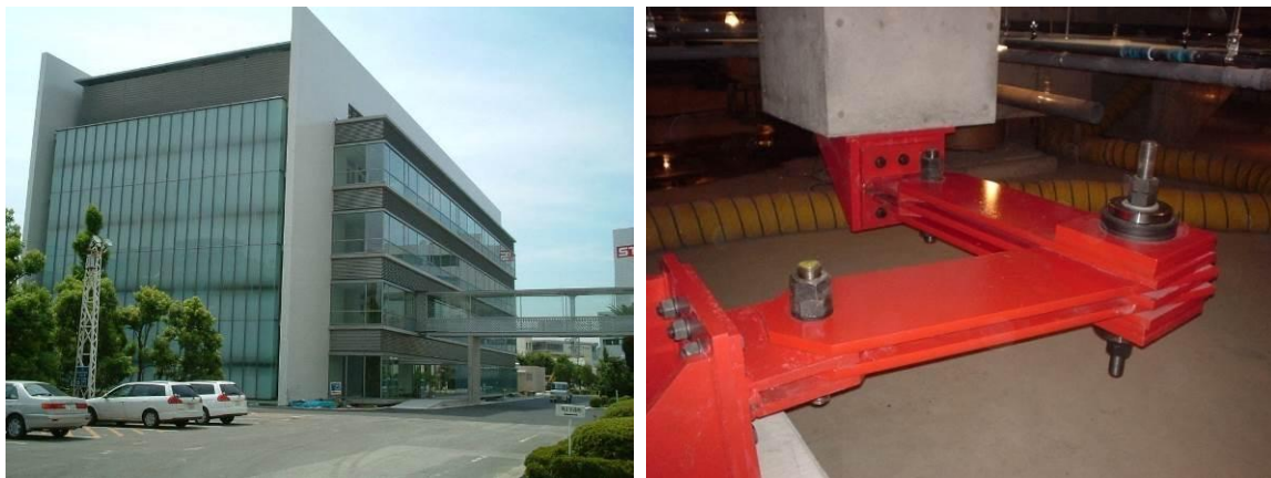
Figure 11 - a: 5 Story Laboratory building. b: Damper installed at the base of the building
