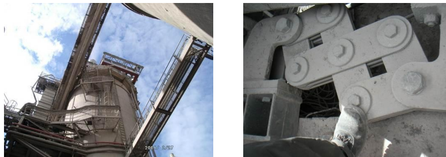
Figure 8 – Scissor Dampers in Industrial plant in Greece
