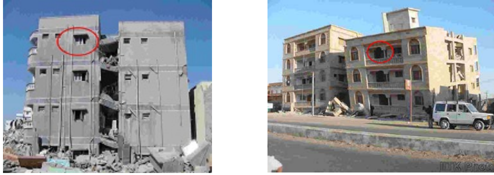
Fig. 1 - Collapse of open ground storey (OGS) RC frame residential building with small to large openings at Bhuj during 2001 Bhuj earthquake [Source: www.nicee.org ]
