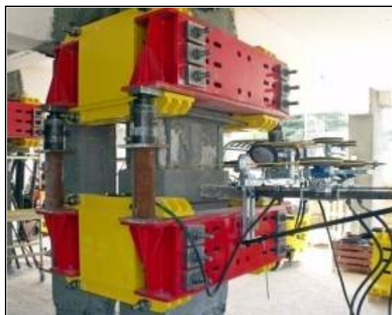
Fig. 19 – Cutting machine with diamond wire
