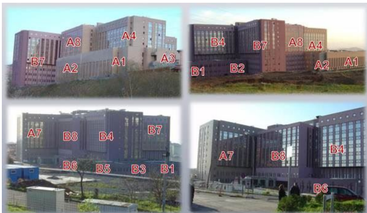
Fig. 2 – View of the different blocks of the building
