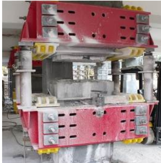
Fig. 20 – Removal of the portion of column
