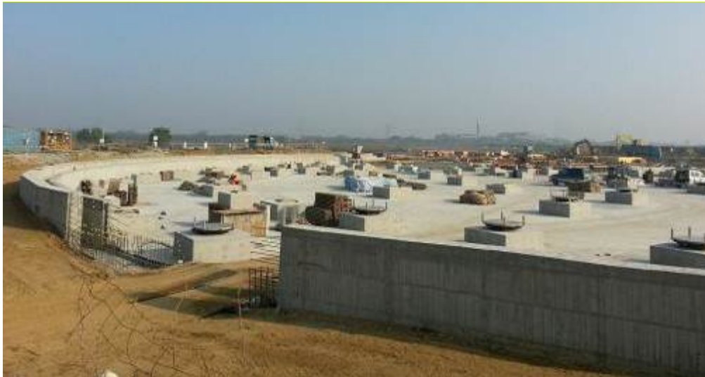
Fig. 11 – General view of the installed sliding pendulum
