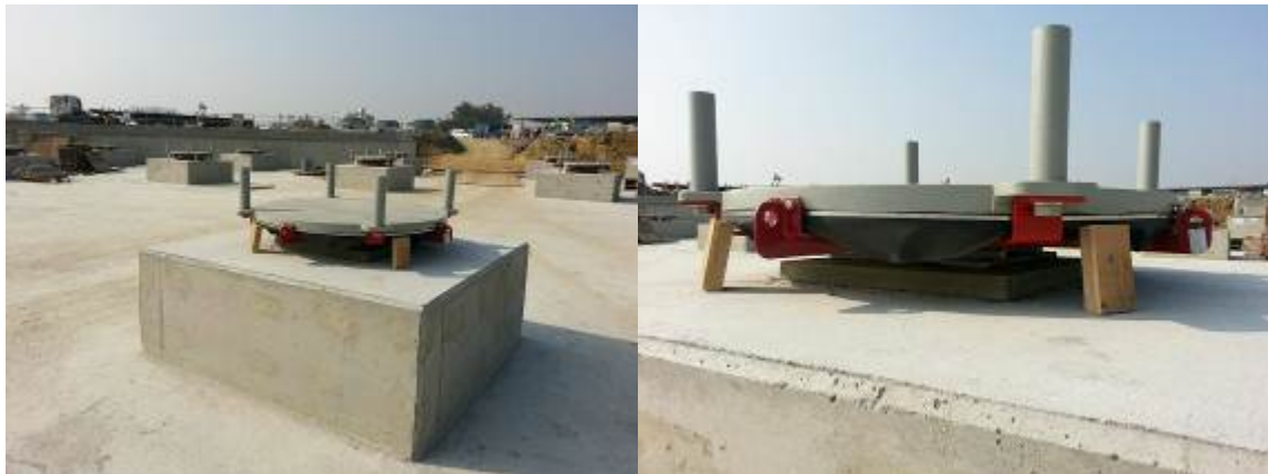
Fig. 10 – Installation of the sliding pendulum before casting the concrete slab
