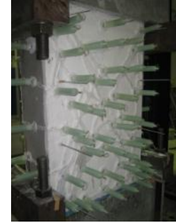
Fig. 8 – Epoxy resin injection
