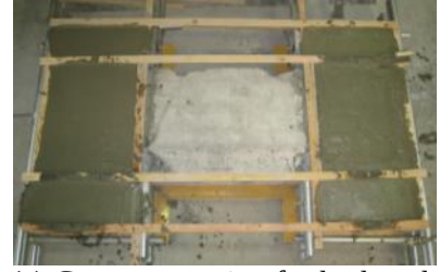
(c) Concrete casting for both stubs
