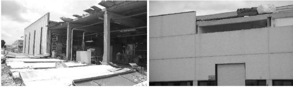
Fig. 2 The collapse of the cladding panels in an industrial precast building (left), and in a commercial building (right), both after the Emilia-Romagna earthquake (2012)
