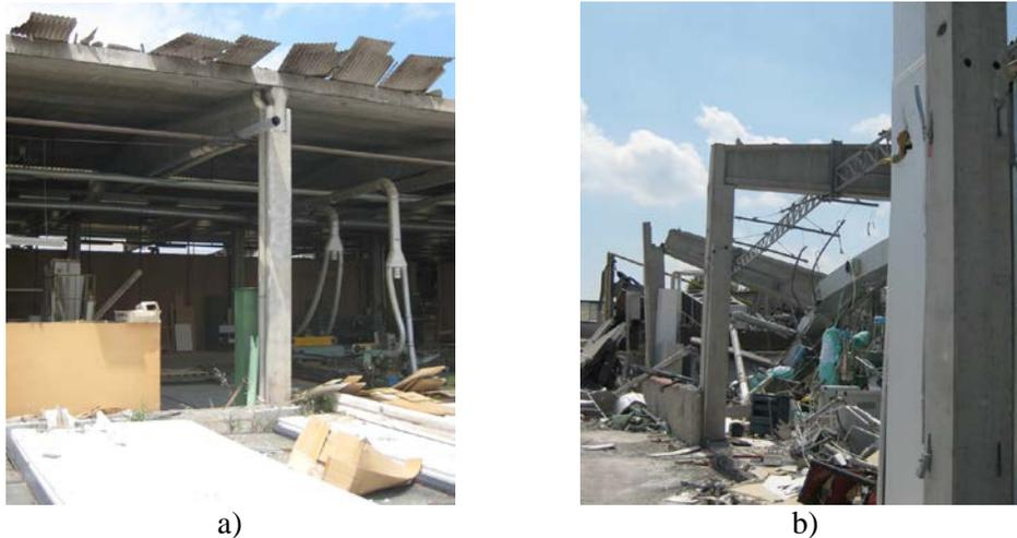
Fig. 1 – a) Dislocation of precast vertical panels, and b) collapse of a precast RC building due to the 2012 earthquakes in the Emilia Romagna region.
