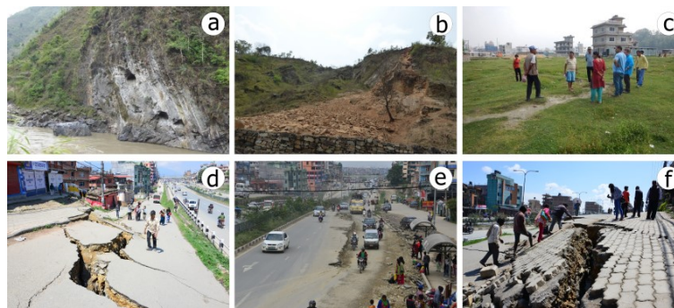
Fig. 3 – Typical EEE induced by the 2015 Nepal, Gorkha earthquake: (a, b) landslides along the road network of the affected area, (c) liquefaction phenomena in Guheshwori from [26] (d, e, f) ground cracks strongly related to liquefaction-induced lateral spreading along a segment of the Kathmandu-Bhaktapur road section of the Araniko Highway in the Lokanthali area.
