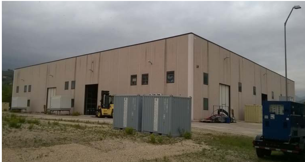
Fig. 1 – The building of the Civil Protection Centre in Foligno, Italy
