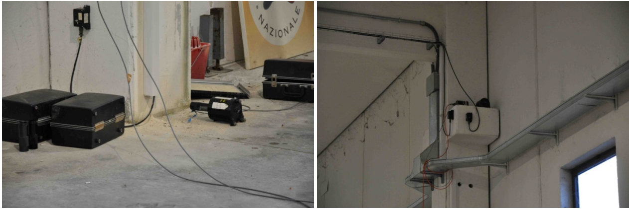
Fig. 5 – Location of accelerometer A11 and seismometer S11 (left) and location of accelerometers A08 and A09 and seismometers S08 and S09 (right) on frame F2.
