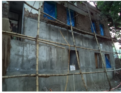
(h) Concreting work on perimeter brick wall
