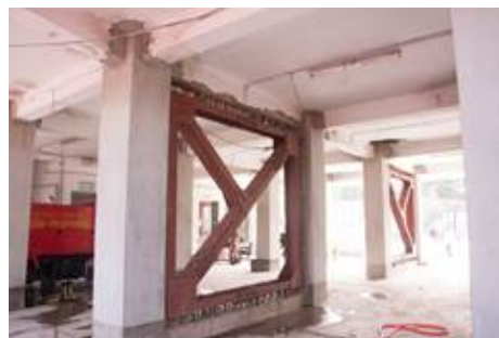
(e) Placing of steel framed brace
