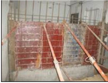
(g) Construction of RC wall at grid -4
