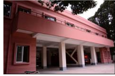
(i) New look of fire station building after retrofitting
