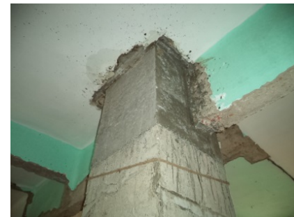
(c) Non-shrink grout mortar work at top of column, 1 st story
