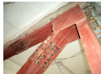
(f) Connection of steel framed brace
