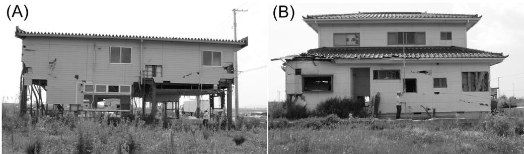
Fig.2 Examples of destroyed and undestroyed building side walls: (A) destroyed and (B) undestroyed.
