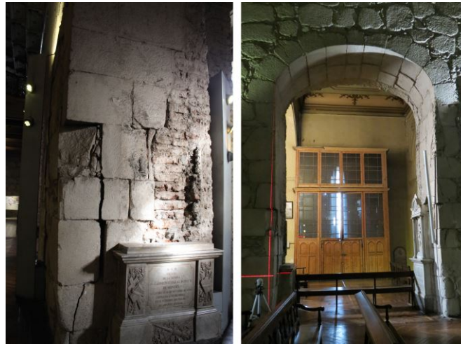
Fig. 3- Deformation of an arch and dangerous cracks in its base.
