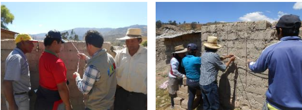
Figure 10 – Practical training in the nylon-rope mesh technique
