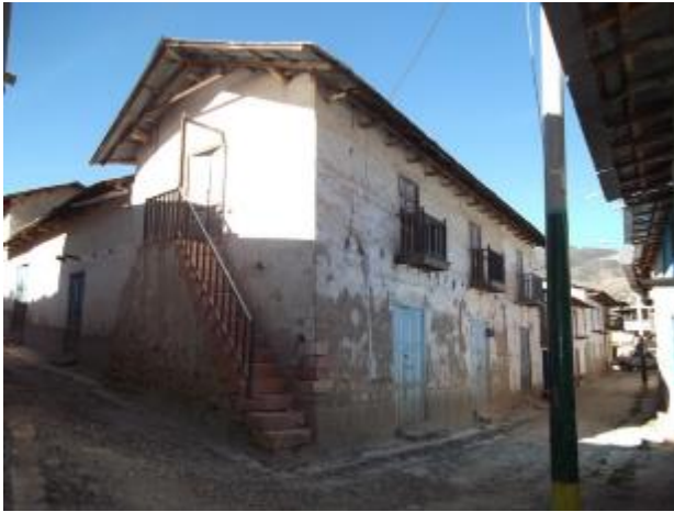
Figure 8 – A typical two-story adobe house in Pullo
