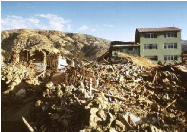
Figure 1 – Destroyed adobe houses (Huaraz, 1970) (credits: Vargas et al. 2005)
