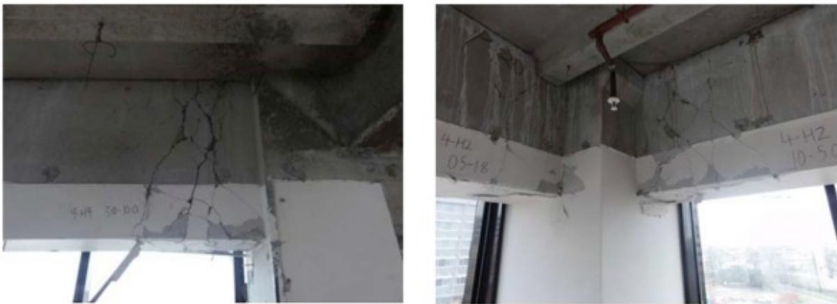
Fig. 1 Beam plastic hinges in a 22-storey reinforced concrete building constructed in mid-end 1980s [3].
