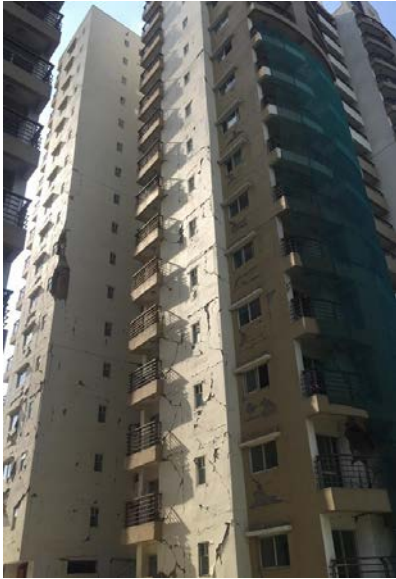
Fig. 11 Exterior cracking, residential tower
