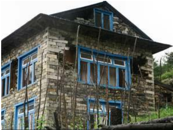
Fig. 9 Out-of-plane failure of bearing wall building
