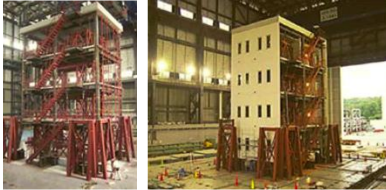
Fig. 1 – Steel frame tested at E-Defense.
