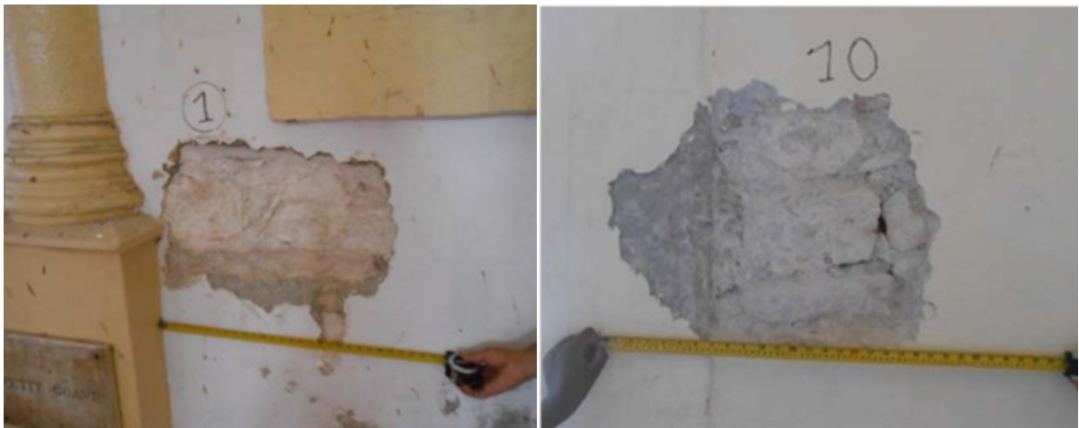
Irregular-shaped stones placed in the mortar Rectangular-shaped stone and debris in mortar Fig. 7 Typical composition of exposed unreinforced masonry stone walls
