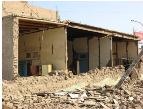
Fig. 1 - Damage of adobe houses during the Pisco (Peru) earthquake of 2007
