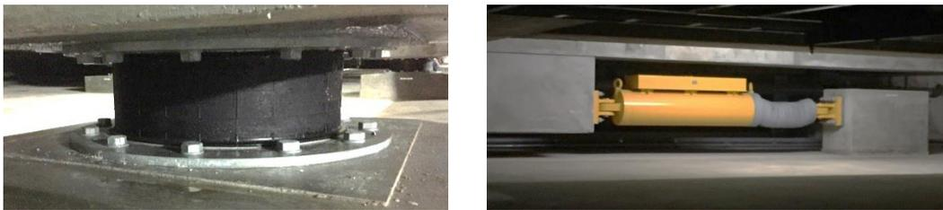
Fig. 1 – Hybrid base-isolation system on the campus of Tohoku University.
