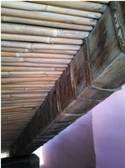
Fig. 5 (left) – Leather lashing of beams with reed sheathing under eave, photo by author
