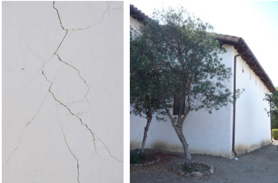
Fig. 11 (left) – Displacement markings on east Sacristy wall, photo by author
