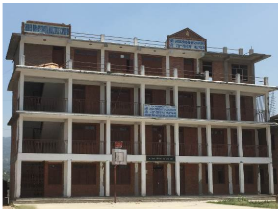
(a) west elevation view
