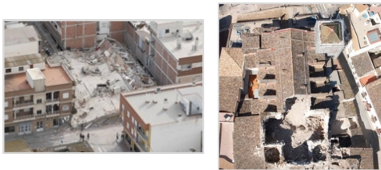
Fig. 1 – Typical damage. Left: collapsed building. Right: collapsed roof and cupola of the church known as “ Iglesia de Santiago ”.
