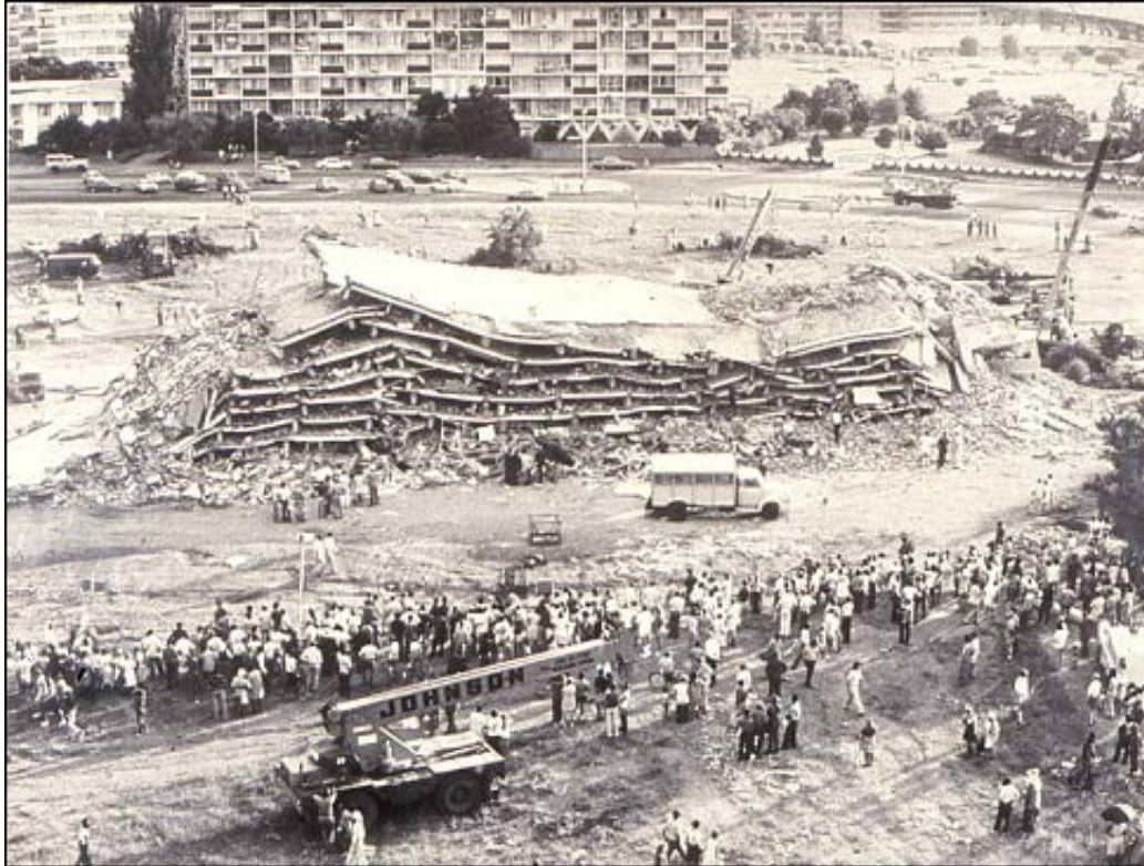
Fig. 1 – Dramatic photograph of a collapsed residential building in Welkom (South Africa) after a strong rockburst with local magnitude M_L=5.2 , from December 8 th 1976 (courtesy of Dr A. Cichowicz, South African Council for Geoscience).
