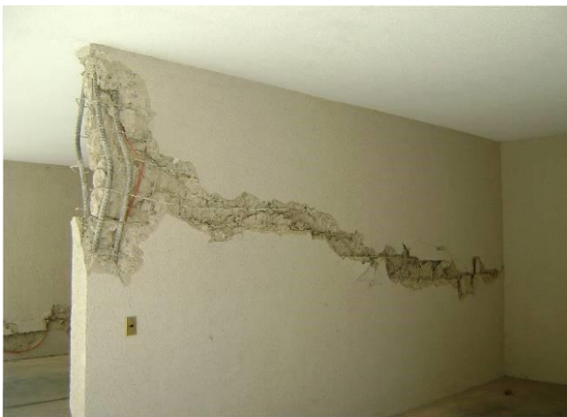
Fig. 1 – Damaged web of a T-shaped wall and a plane of the 1 st story with the most important damages
